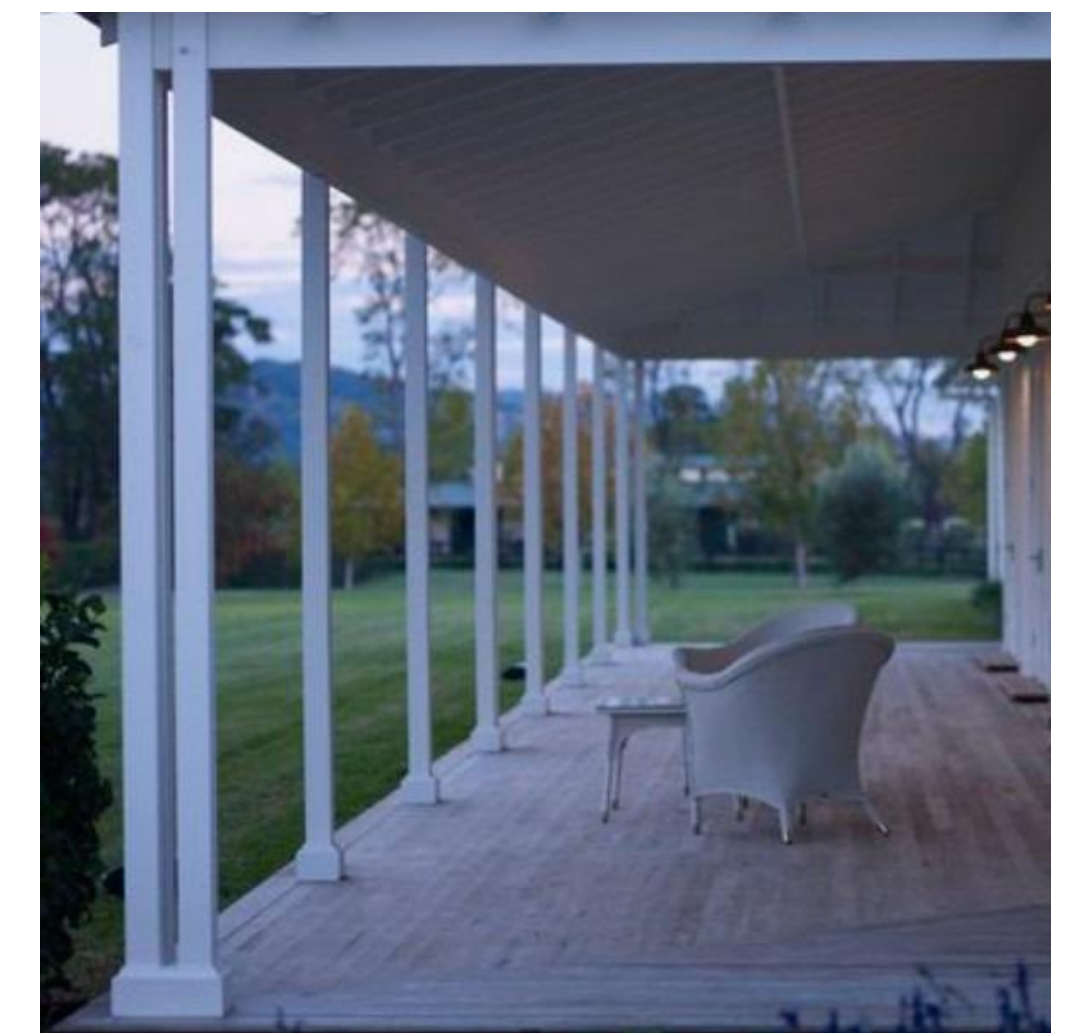
PAINTED VERANDAH POSTS
